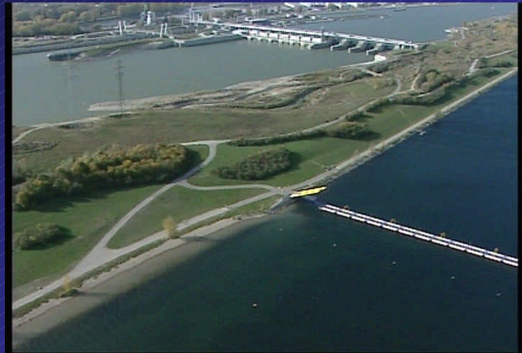
Hydropower Plant Freudenuau
